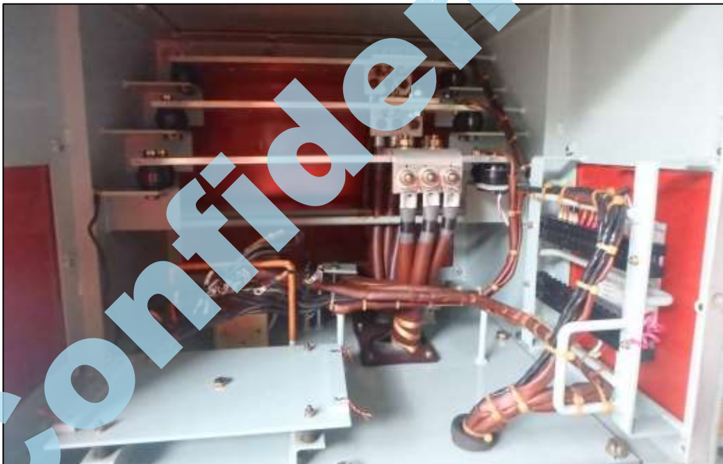
Fig. 26 & 27: Condition of LH space heater and RH space heater after re-installed as per original.
