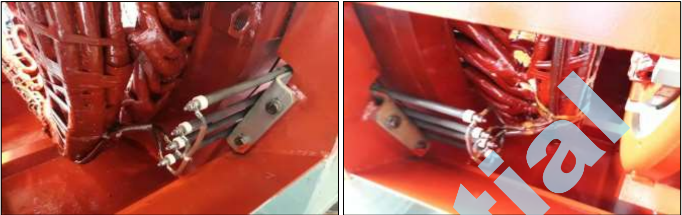
Fig. 26 & 27: Condition of LH space heater and RH space heater after re-installed as per original.
