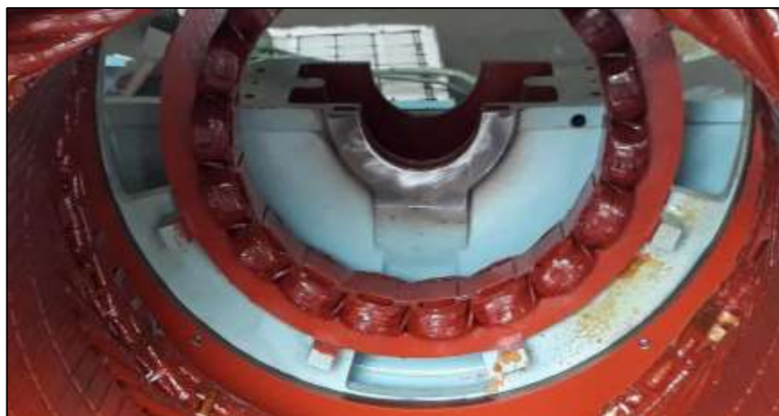
Fig. 21 & 22: Condition of Lower part bearing housing after re-installed.
